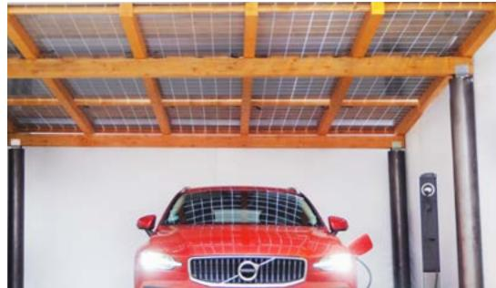
Solid structural timber on columns made of special steel
