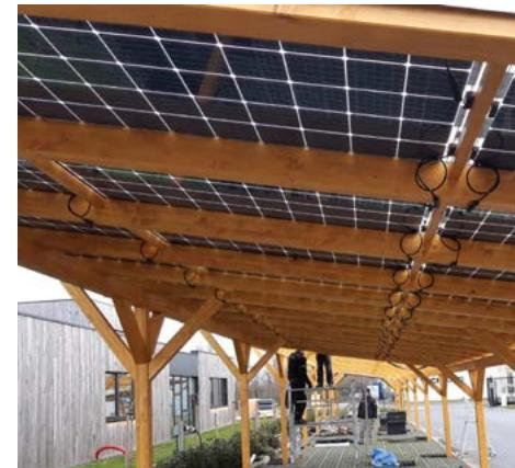
**stable wooden construction in combination with transparent double glass modules**
