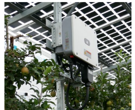
Safe mounting of inverters
